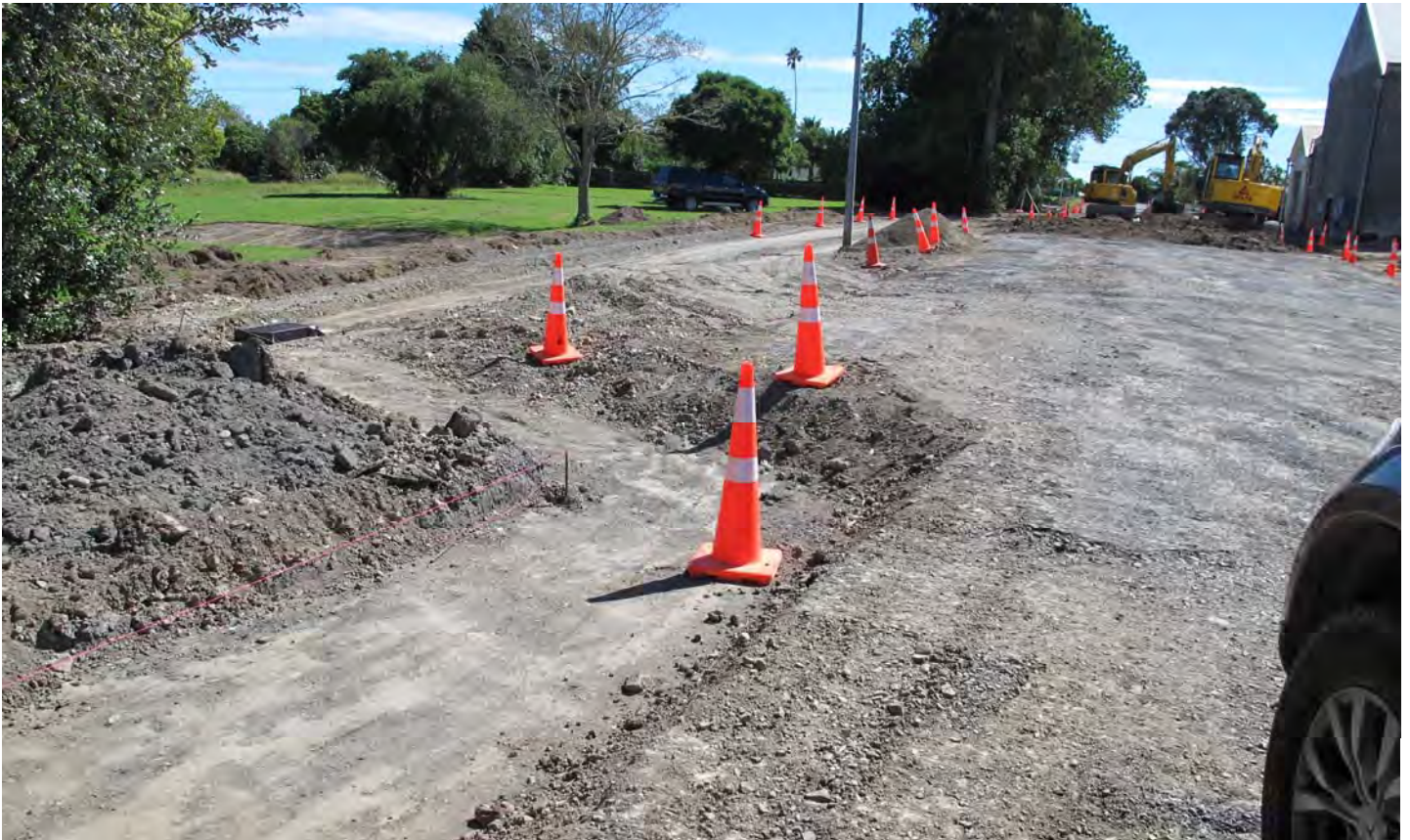
Image: Contractors work on installing new footpath, curb and channel and parking in Potts Ave as part of our Asset Renewal programme.
