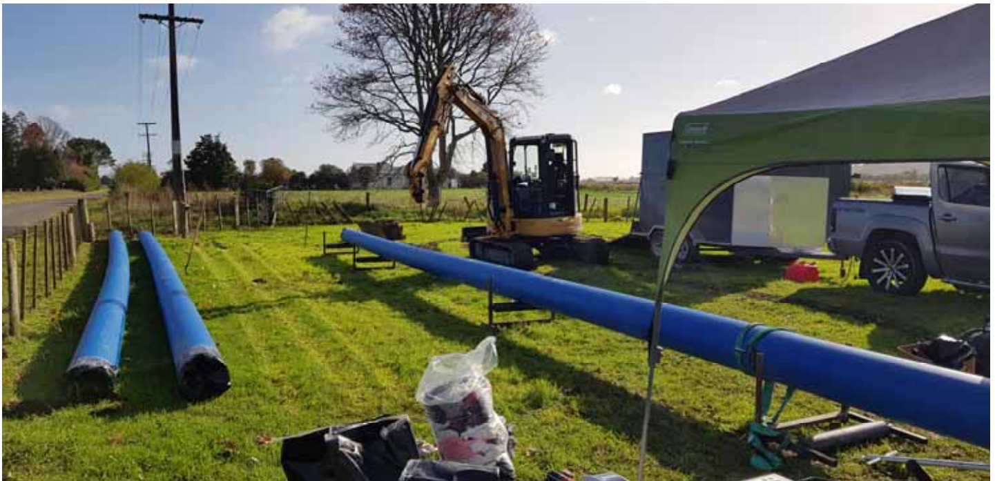
Image: Welding of pipes to replace the ageing raw water supply main along Otara Road from Clarks Cross Road to the pump station is in progress.
