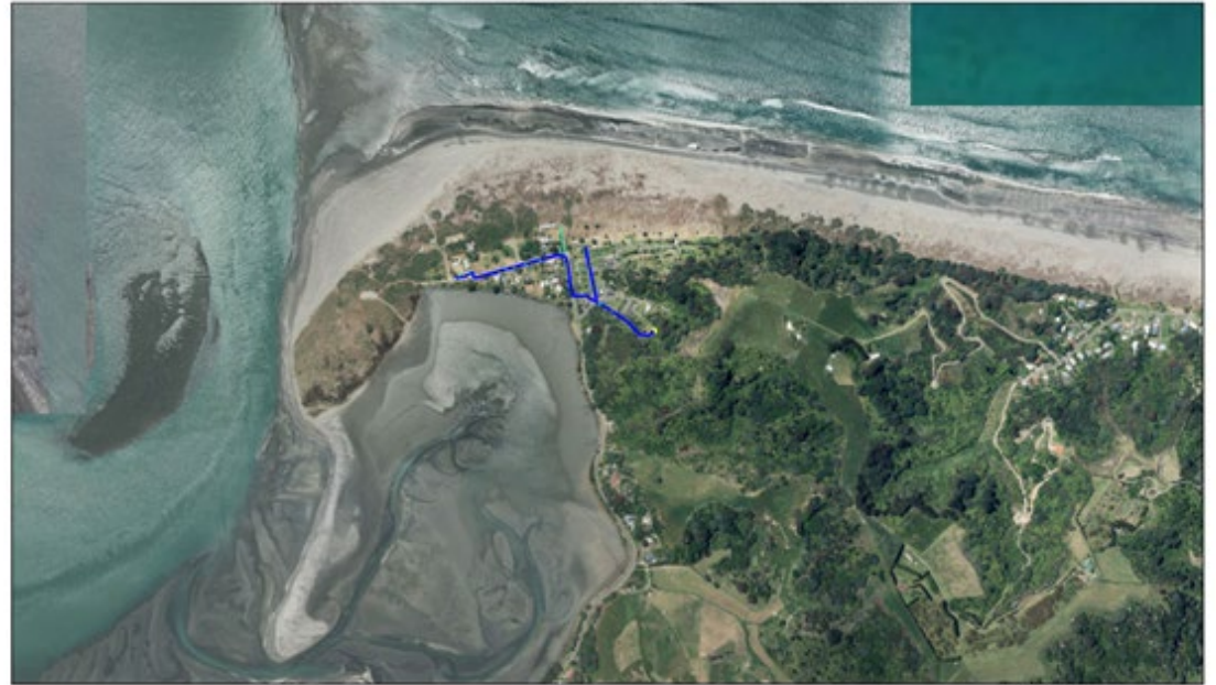
Ohiwa Water Supply Area
