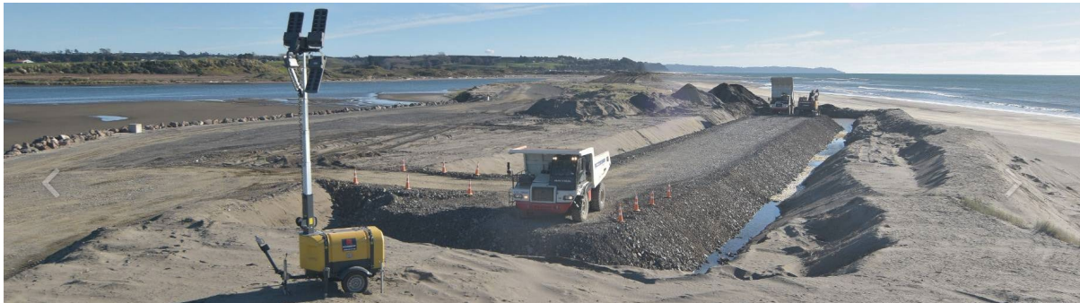
Figure 6-1: Construction progress of the eastern training wall May 2021 (Source: HEB Construction)
